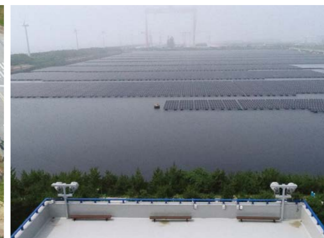
Gunsan Floating solar facilities Light Level : 15LUX Fixture : LED 1200W (Q'ty:4) Pole : 3m (Q'ty:2)
