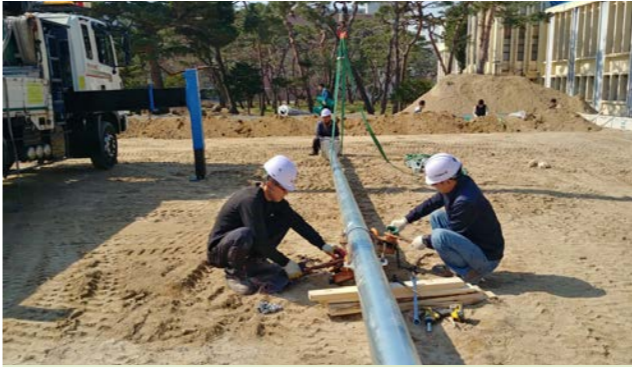
5. Pole assembly / assembly of lighting fixture and converter box
