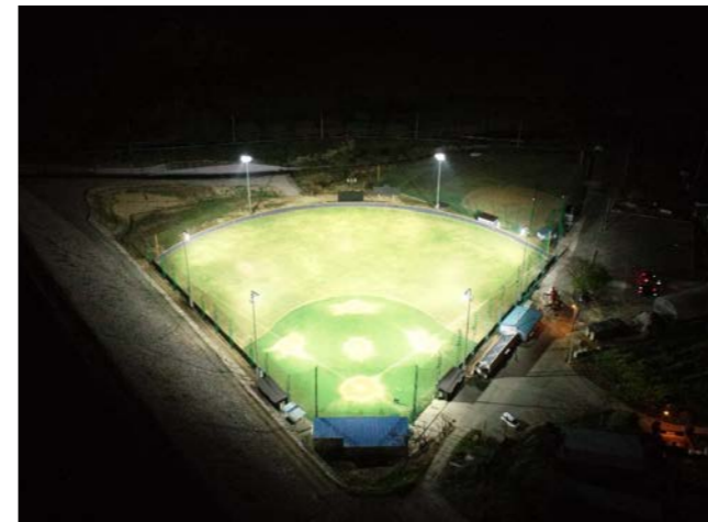
Hampyeong Jeonnam Baseball Light Level : infield 800LUX outfield 500LUX Fixture : LED 1200W (Q'ty:64) Pole : 27m(Q'ty:4), 25m(Q'ty:2)
