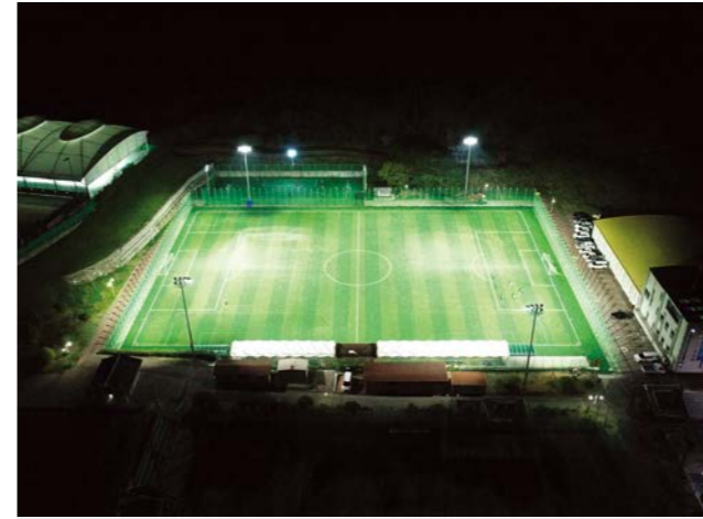
Haenam Usul Stadium [auxiliary stadium] Light Level : 500LUX Fixture : LED 1200W (Q'ty:32) Pole : 21m (Q'ty:4)
