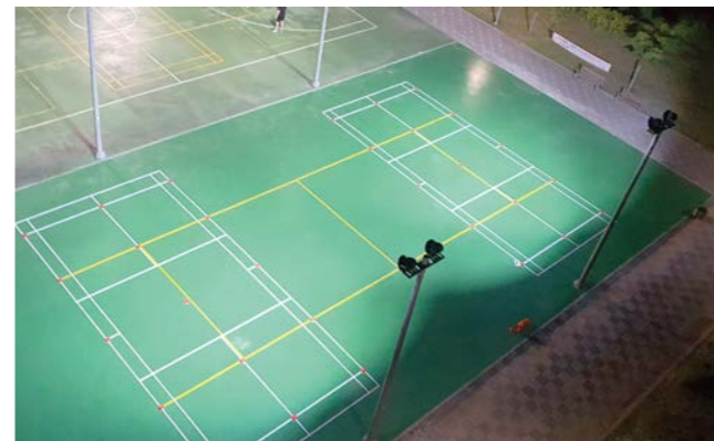
Gimpo Masandong Multi-field Light Level : 200LUX Fixture : LED 300W (Q'ty:4) Mounting Height : 8m
