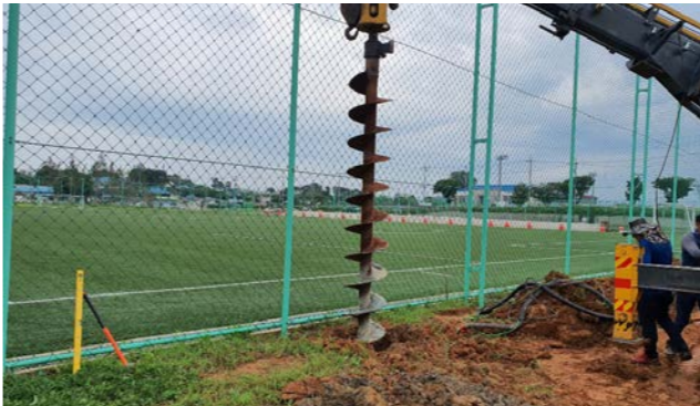
1. Foundation perforation
