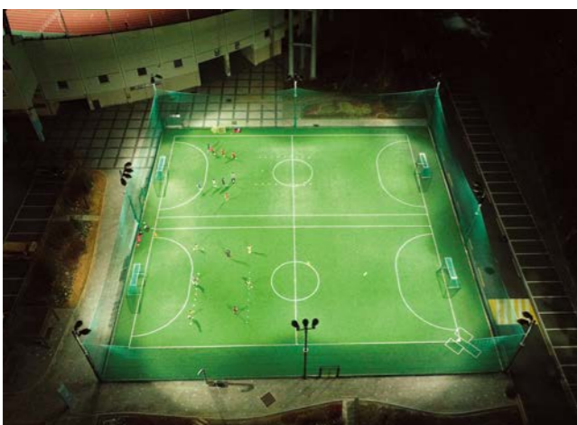
Mokdong Sports Complex Multi-Field Light Level : 500LUX Fixture : LED 600W (Q'ty:22) Pole : 10m (Q'ty:8)
