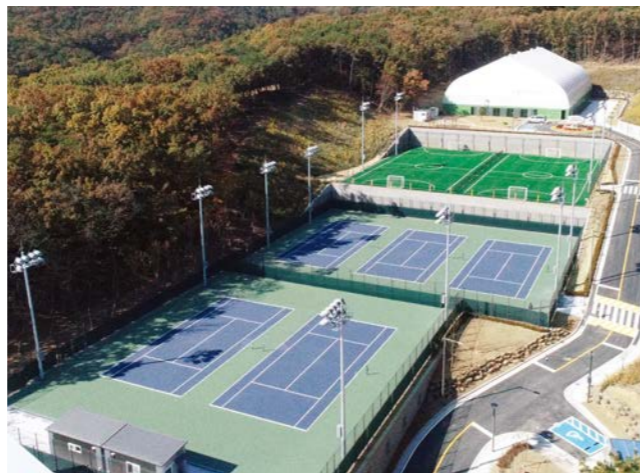
Gimpo Seoam Sports Park [indoor&outdoor] Light Level : indoor 400LUX & outdoor 500~1250LUX Fixture : LED 600W (Q'ty:84) & LED 200W (Q'ty:24) Pole : 15m (Q'ty:12)
