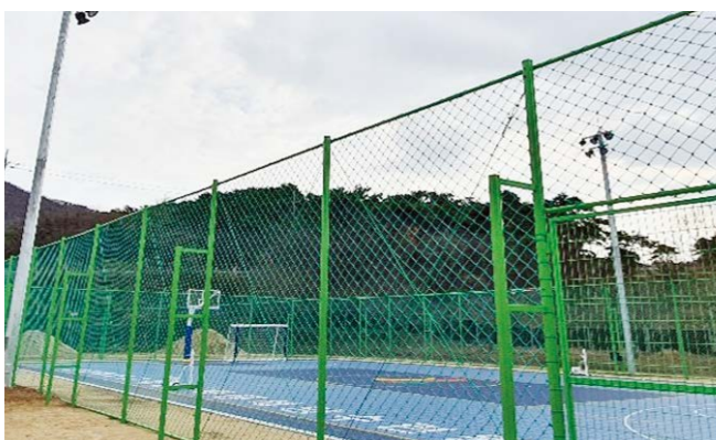
Jeonbuk Student Marine Training Center Futsal Light Level : 250LUX Fixture : LED 300W (Q'ty:12) Pole : 9m (Q'ty:2)
