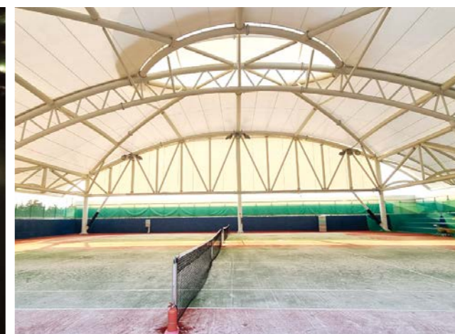
Muan Sports Park Tennis Court Light Level : 850LUX Fixture : LED 600W (Q'ty:18) Mounting Height : 10~12m
