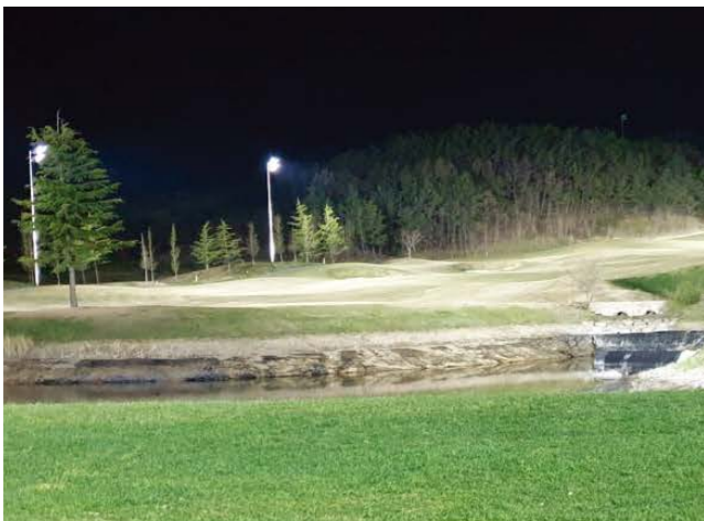
Ocean Hills Cheongdo G.C. Light Level : 200-150-350LUX Fixture : LED 1200W (Q'ty:35) Pole : 15m (Q'ty:11)
