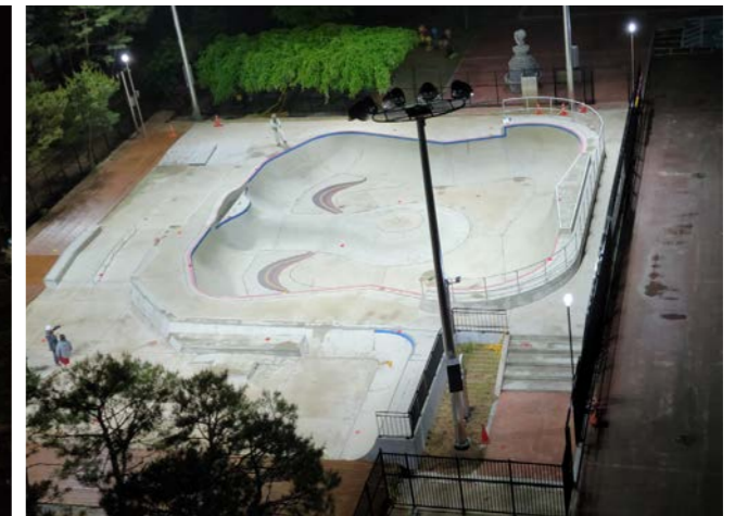
Andong Extreme Park Light Level : 800LUX Fixture : LED 600W (Q'ty:16) Pole : 12m (Q'ty:4)
