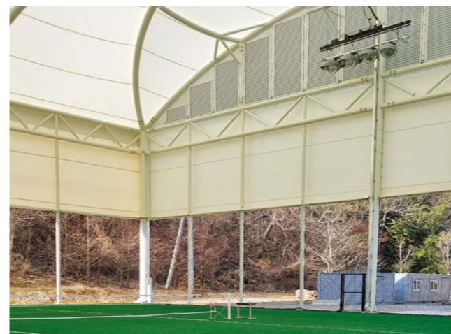
Naju Jokgu Light Level : 400LUX Fixture : LED 600W (Q'ty:8) Mounting Height : 14m
