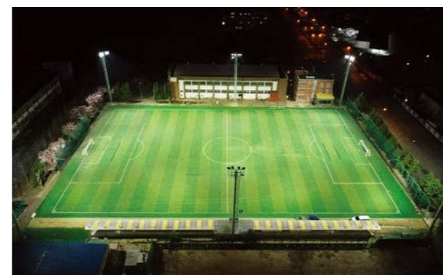
Jeonju Technical High School Soccer Field Light Level : 500LUX Fixture : LED 1200W (Q'ty:46) Pole : 25m (Q'ty:6)
