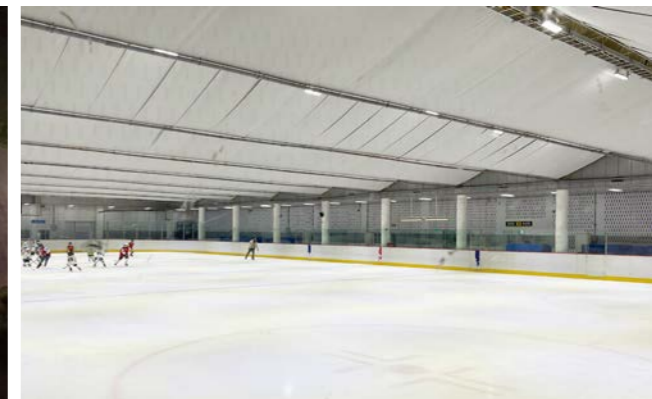
Mokdong Ice Rink Light Level : 1000LUX Fixture : LED 200W (Q'ty:75) Mounting Height : 6m
