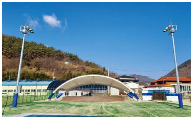
Nonsan Beolgok-myeon Multi-Field Light Level : 50LUX Fixture : LED 600W (Q'ty:6) Pole : 12m (Q'ty:2)
