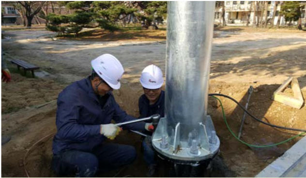
7. Foundation+pole assembly
