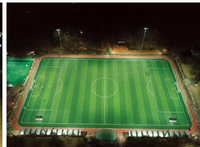
Wonju Dangwan Soccer Light Level : 150LUX Fixture : LED 1200W (Q'ty:20) Mounting Height : 21m
