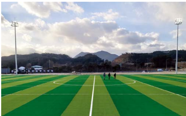
Chunhyanggol Sports Park Soccer Field Light Level : 600LUX Fixture : LED 1200W (Q'ty:48) Pole : 24m (Q'ty:4)
