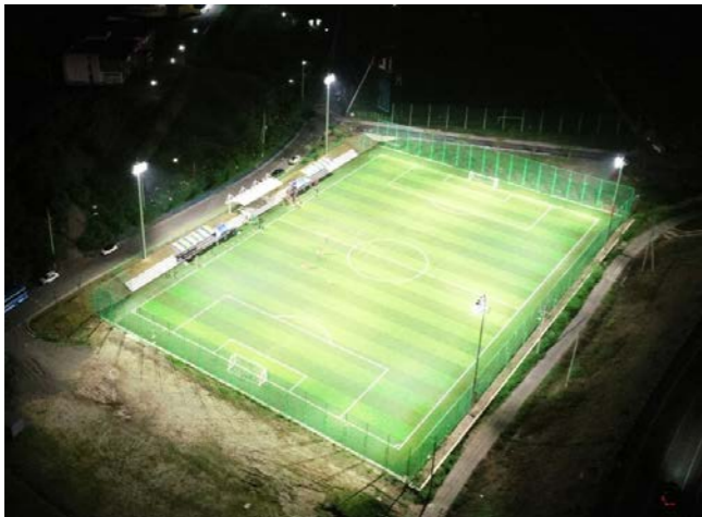
Jangheung Jeongnamjin Resort Soccer Light Level : 600LUX Fixture : LED 1200W (Q'ty:48) Pole : 24m (Q'ty:4)
