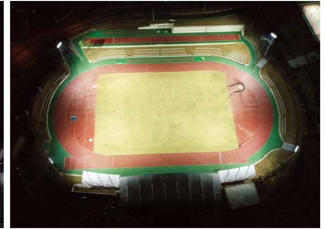
Geumsangun Sports Complex Light Level : 400LUX Fixture : LED 1200W (Q'ty:70) Pole : 27m (Q'ty:4)
