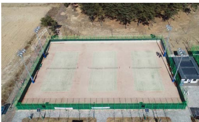
Yecheon New Town Tennis Court Light Level : 950LUX Fixture : LED 1000W (Q'ty:20) Pole : 15m (Q'ty:4)
