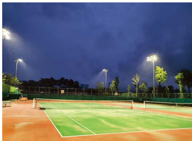
Sejong Water Quality Restoration Center A Treatment Plant Tennis Court Light Level : 700LUX Fixture : LED 1000W (Q'ty:24) Pole : 15m (Q'ty:8)
