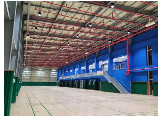
Yeosu Jinnam Badminton Light Level : 1000LUX Fixture : LED 400W (Q'ty:45) Mounting Height: 11m
