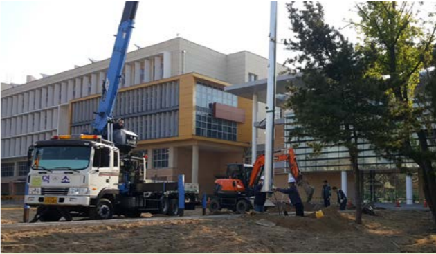
6. Pole erection
