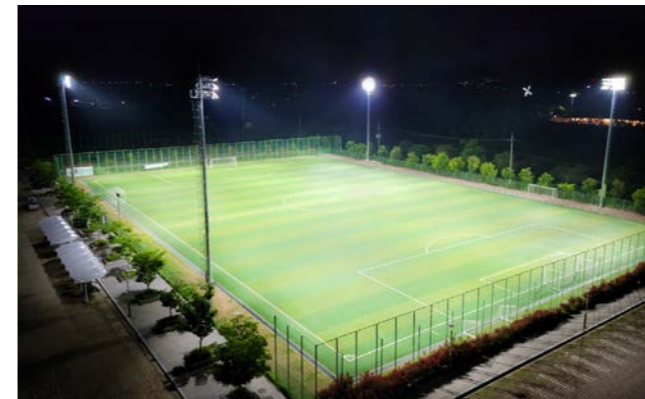
Suncheon National Garden A-Soccer Light Level : 800LUX Fixture : LED 1200W (Q'ty:60) Pole : 25m (Q'ty:4)
