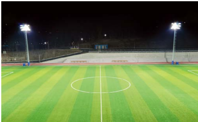
Suncheon Palma Auxiliary Soccer Light Level : 200LUX Fixture : LED 1200W (Q'ty:24) Mounting Height : 25m
