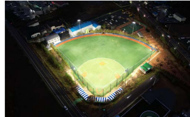
Yeongwol Baseball Light Level : infield 800LUX outfield 500LUX Fixture : LED 1200W (Q'ty:50) Pole : 25m (Q'ty:6)
