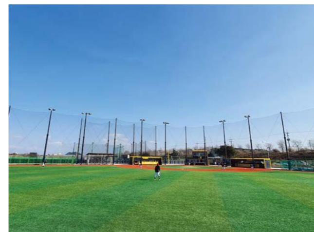
Gangneung Little Baseball Light Level : infield 600LUX outfield 300LUX Fixture : LED 1200W (Q'ty:24) Pole : 15m
