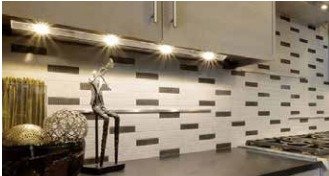
Surface mounted on cabinets
