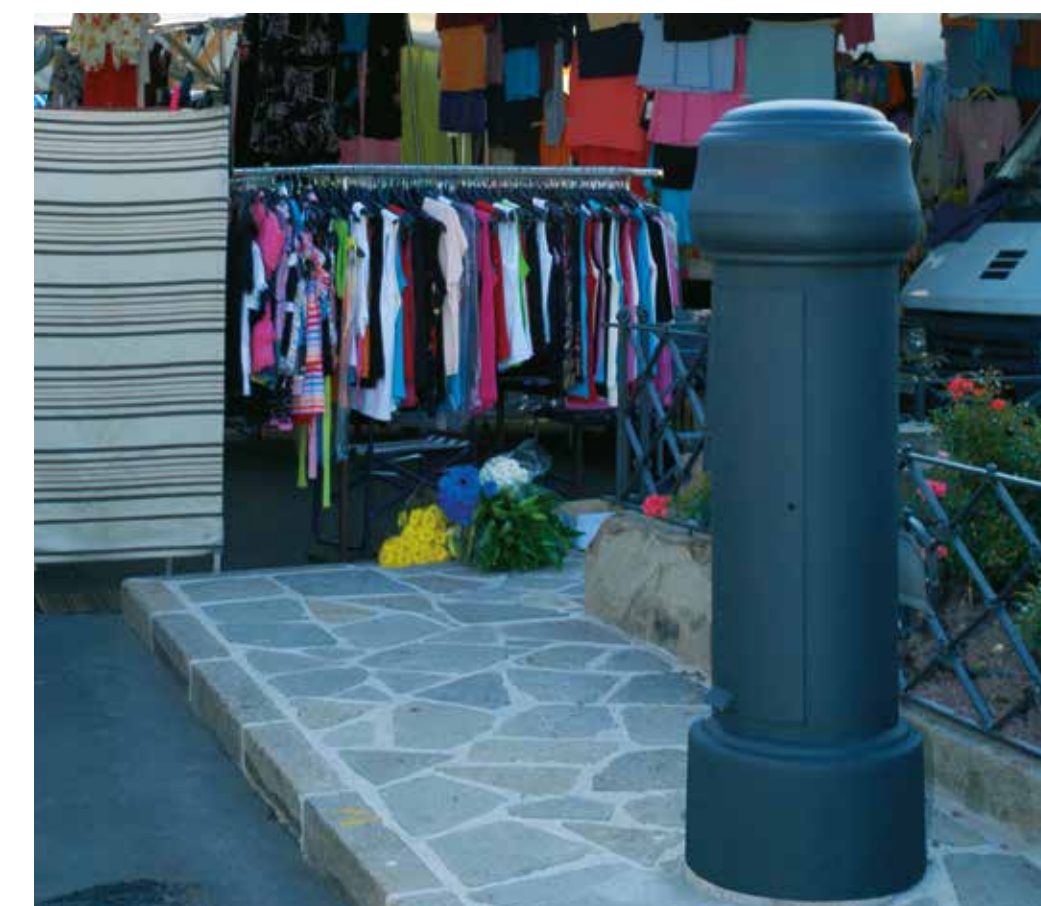
Electricity feeder pillar
