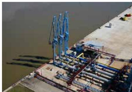
Special oil feeders must balance the filling level of the tanker as it can drop down up to 18m. The capacity of the anchoring area where the fuelling takes place is 8,000 - 12,000 m<sup>2</sup> / hour.
