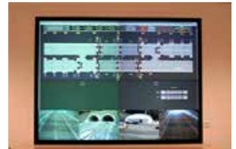
The control (dispatch) room is equipped with two full-size computer workstations and with a graphic screen of the Police of the Czech Republic. This screen is used to control the traffic in the tunnel as well as the technology in the tunnel using Tecomat PLC - 25 km away. Monitoring and control functions are created in Reliance SCADA / HMI system.
