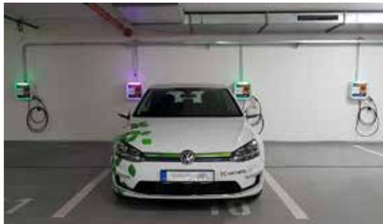
Each parking space in the Moneta underground car park is equipped with a charger. The status of the charger is indicated by coloured LED indicator. All chargers are connected by a two-wire CIB bus and Foxtrot controls them online while using a cycle time of up to 150 ms. Thirty six charging stations available now are to be expanded in the near future and shall reach more than 100 stations.
