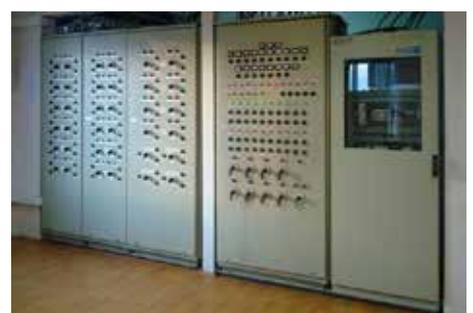
Typical set of 2 switchboards for 4 tanks with the relevant group of automatically controlled valves.
