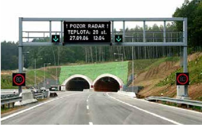
The Valík tunnel together with the adjacent bridge over the Úhlava river is the last section of the motorway which bypasses the city of Pilsen and the D5 motorway from Prague to Rozvadov. The control system has been designed for this tunnel - the first one in the Czech Republic, and the project was completed using two domestic products - our Tecomat control system and Reliance SCADA / HMI system.
