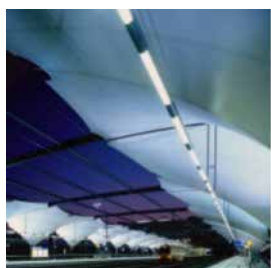
Airport Halle/Leipzig IC station
