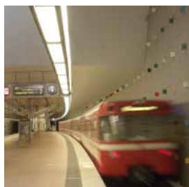
Fürth: Metro station Stadthalle
