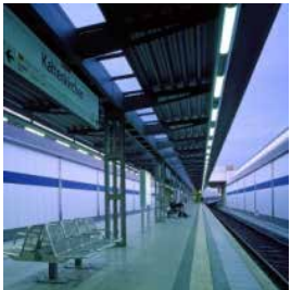
Kaltenkirchen: AKN station
