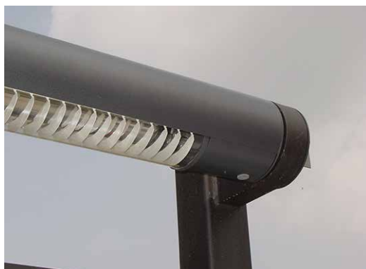
Lighting tube at the baffle
