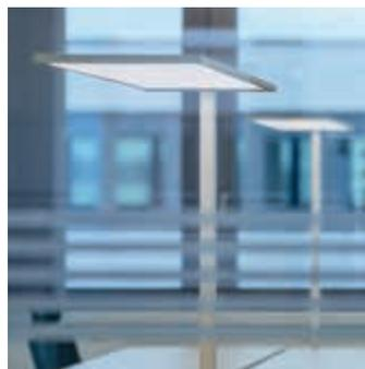
When planning and implementing the lighting concept for the VW subsidiary ITV City, the focus was on the dynamic adaptability of lighting to users, the use of space and lighting requirements. The concept was implemented with over 500 office floor lamps (SL720XL) with daylight controller. The extra-long, only 2 cm high luminaire head ensures standard-compliant illumination of two computer workstations, while the functional U-shaped base enables flexible and simple positioning of the light.
