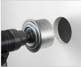
Create installation opening  $\varnothing$  68 mm with KAISER cutter (e.g. MULTI 2000 HM, Art.-No. 1083-70).
