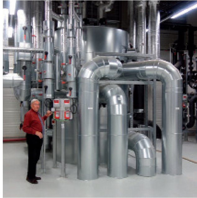
Zortström Multi-H 5-stufig Durchmesser 2.200 mm
