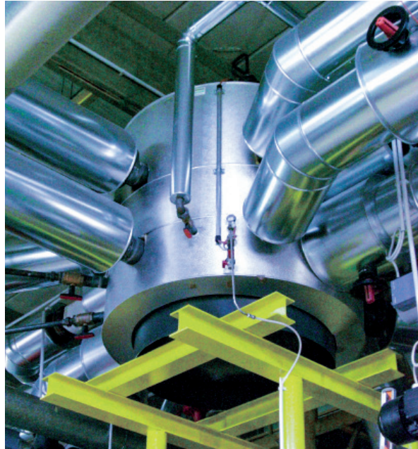
Zortström Multi-H 2-stufig Durchmesser 900 mm
