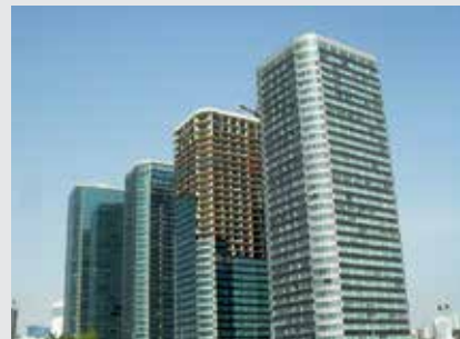
Bahia Center Residential Estate, Oran, Algeria
