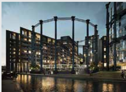
King Cross T1 Building, London, United Kingdom
