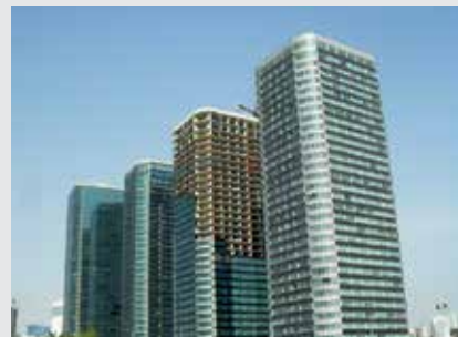
Bahia Center Residential Estate, Oran, Algeria
