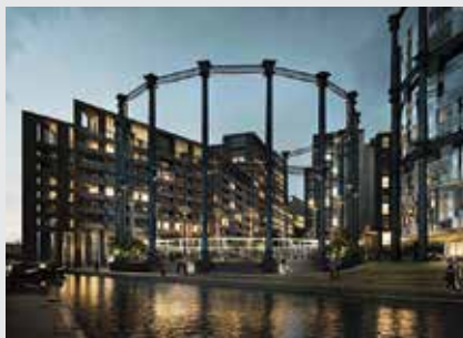
King Cross T1 Building, London, United Kingdom
