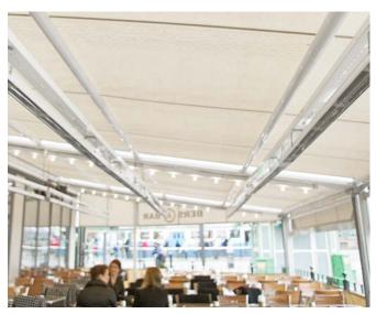
CIR is an ideal solution for giving comfort to customers at outdoor restaurants. The heaters can be mounted on the restaurant's wall or in line directly above the tables in large terraces.
