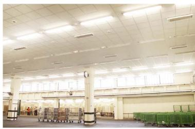
With radiant heaters, the heat is transferred to surfaces such as people, floors and fixtures. This creates comfort even in rooms with large volume.
