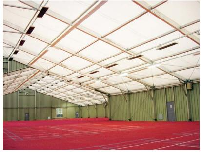
EZ300 gives instant heat and no preheating is necessary which makes it ideal for buildings that are used on an irregular basis.
