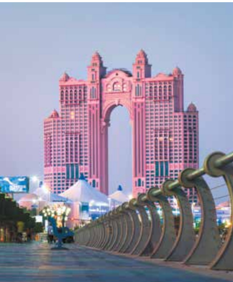
FAIRMONT HOTEL DUBAI - UAE - 2012 Heating/cooling system
