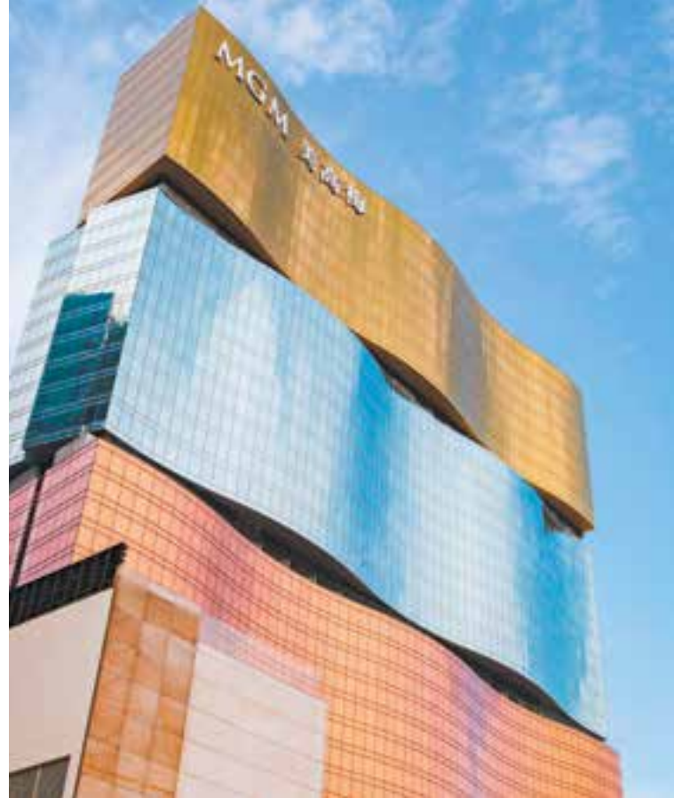
MGM HOTEL MACAU – CHINA – 2017 - Heating/cooling system
