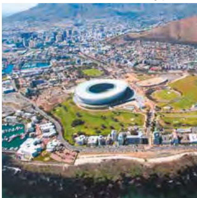
CAPE TOWN STADIUM SOUTH AFRICA - 2009 - Cooling system
