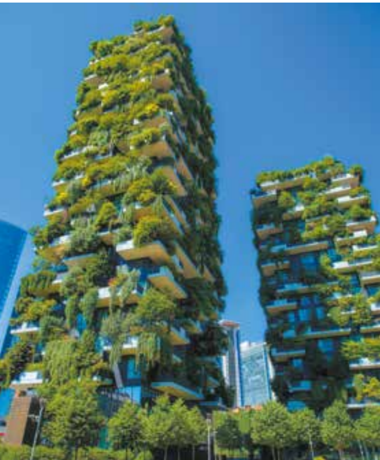
BOSCO VERTICALE MILANO ITALY - 2013 Heating/cooling system
