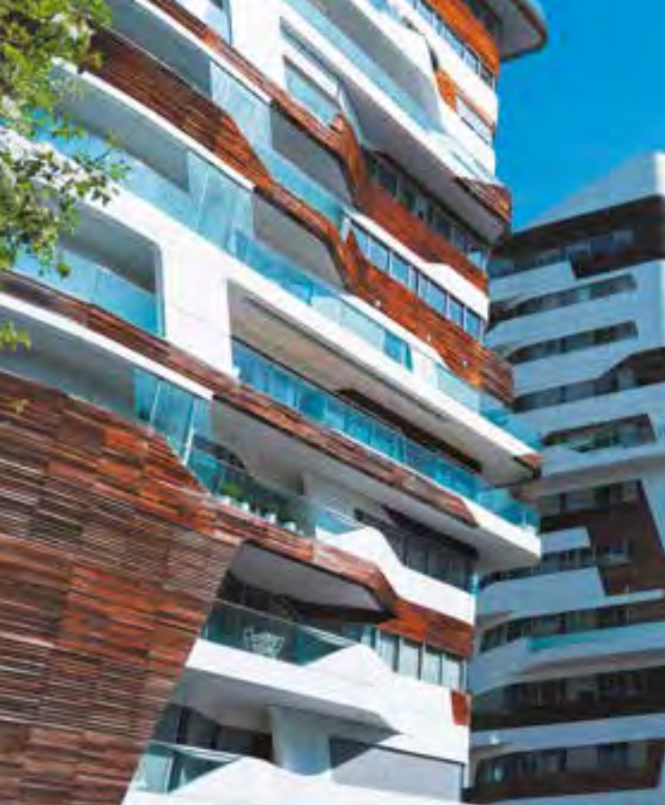
CITY LIFE MILANO ITALY - 2014 - Central heating/cooling + distribution
