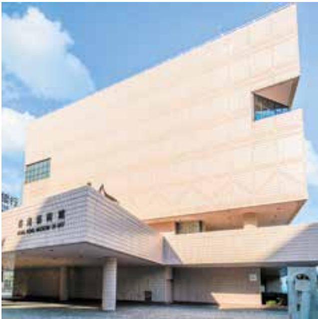
HONG KONG MUSEUM OF ART – HONG KONG CHINA – 2017 - Heating/cooling system
