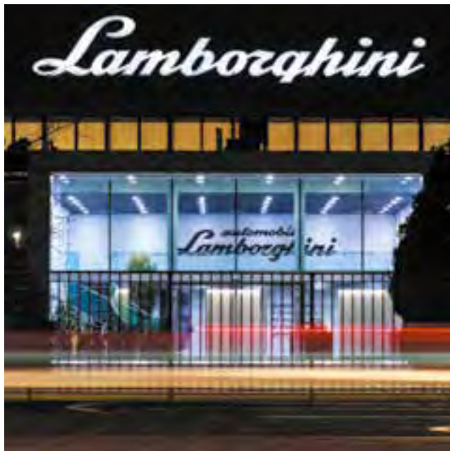
LAMBORGHINI - MODENA ITALY - 2016 Heating/cooling system
