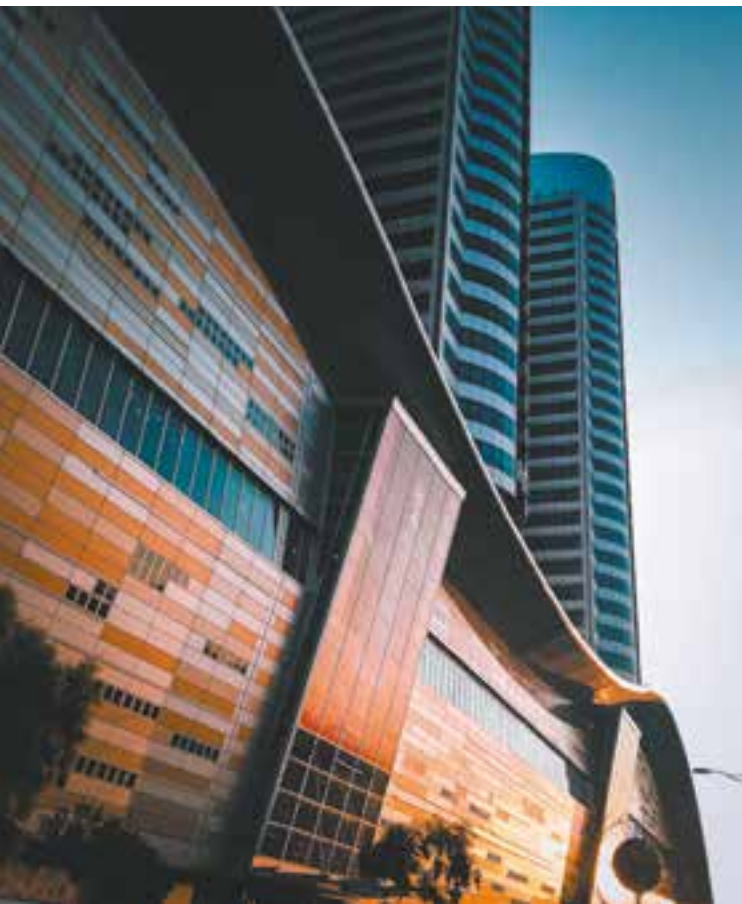
CENTAURUS TOWERS ISLAMABAD PAKISTAN – 2012 - Central heating/cooling + distribution
