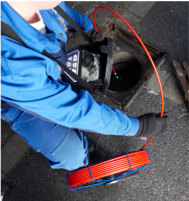
Professionally equipped with camera viper for inspecting underground pipelines.
