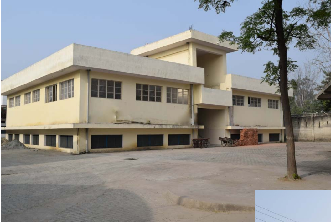
Canteen and Corrugated making area
