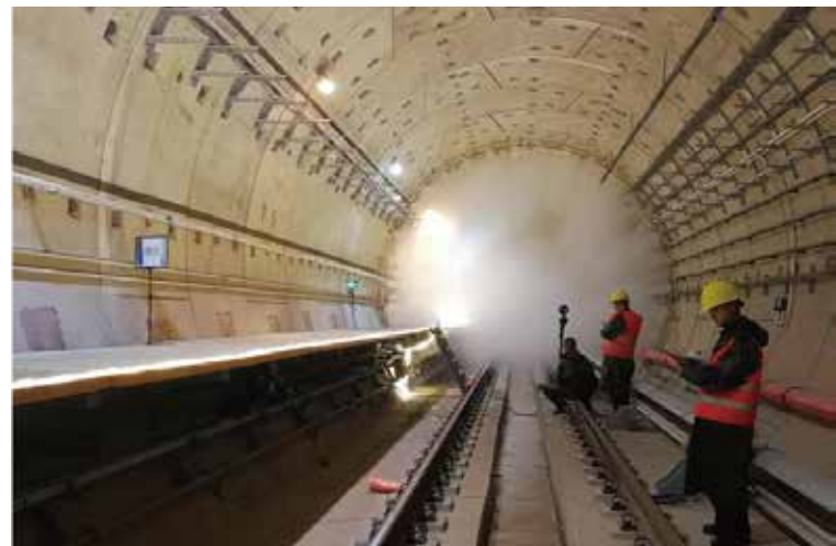
Hangzhou Metro Tunnel Water Mist Curtain
