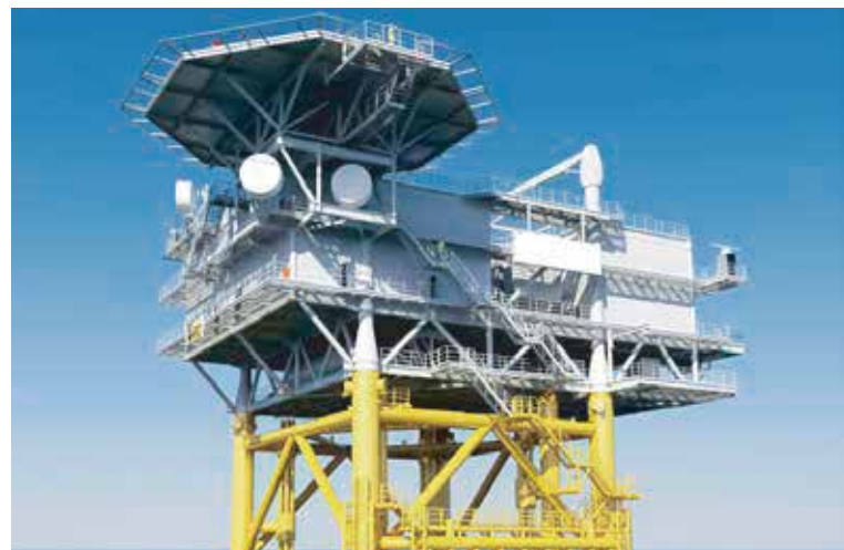
China Offshore Substation
