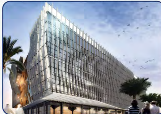
MEDICAL TOWER RIYADH
