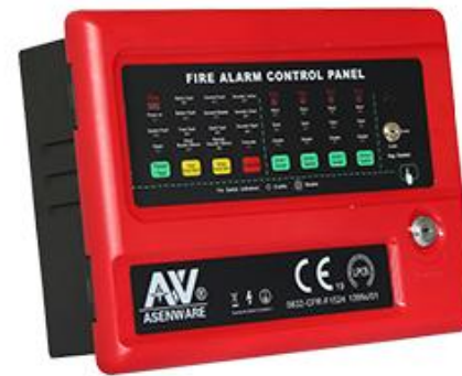
Conventional fire alarm panel 4 zone AW-CFP2166-4
