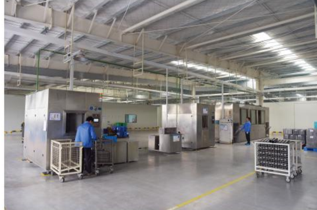
Ultrasonic Cleaning Line
