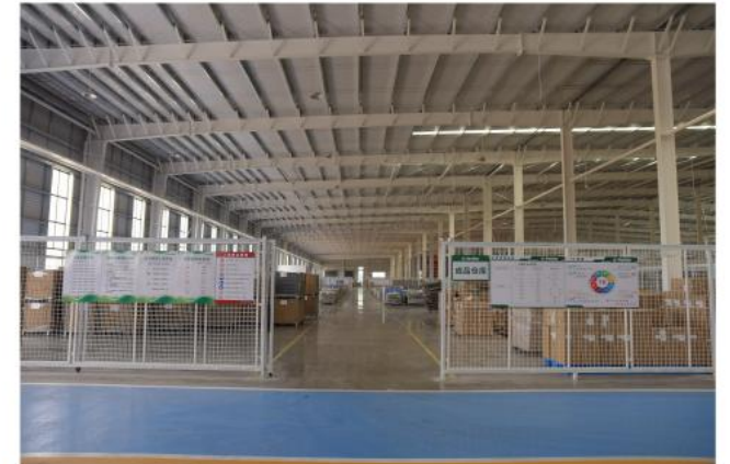
Finished Product Warehouse
