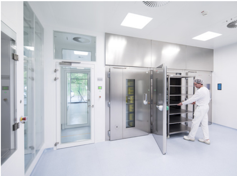
HVS (high velocity streaming) horizontal flow cooling locks for controlled cooling-down of nutritional solutions with integrated temperature and pressure monitoring
