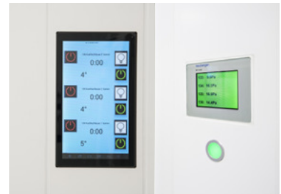
Monitoring of pressure, temperature and humidity in classified cooling locks
