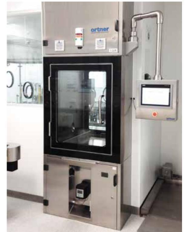
H<sub>2</sub>O<sub>2</sub> decontamination lock in the exit area
