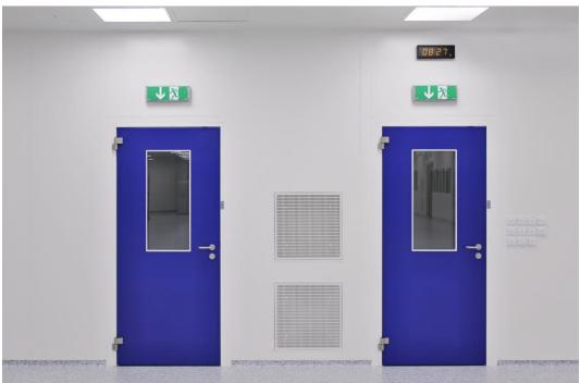
All types of grids and connecting elements are made of stainless steel and are supplied as standard with a surface treatment made with KOMAXIT powder epoxy - polyurethane coating in the shade RAL 9010 semi-matt.
