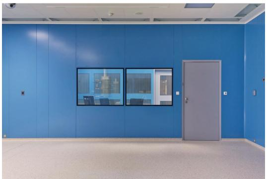
The frame of the EG pharma window is made of steel sheet provided with a powder fired varnish like other elements of ČP. The color solution is usually the same as the shade of the surrounding partition. At the customer's request, painted in any shade, according to the RAL scale.
