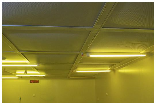
The circulation unit is made of grade 11 steel sheet. The unit has its own self-supporting structure, which is placed on the grid of the laminar field.
