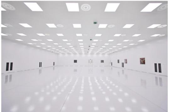
The ceiling is constructed as a raster structure. In the case of using an alternative grid size, the components can be placed in the ceiling by adjusting the grid in a given location or installing the component in cassettes. The grid construction enables the operative rearrangement of suspended ceiling elements in the future according to the needs of newly installed technologies.
