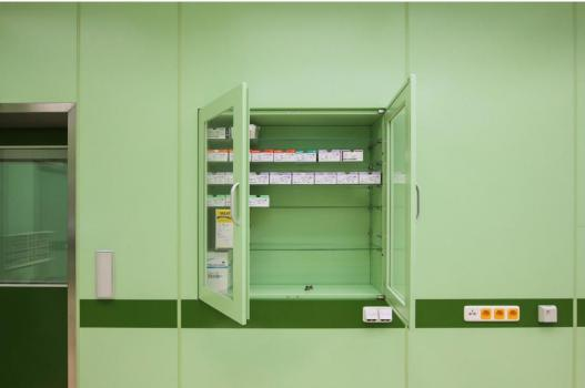
The sewing cabinet is made of RUBACOLOR sheet metal or steel sheet with a surface treatment with powder fired varnish in RAL shade. Shelves can be made of glass, stainless steel or plastic (PE, PVC).
