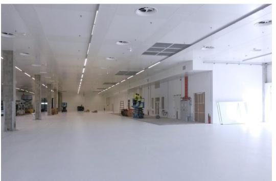
The integrated ceiling EG type ISU consists of supporting aluminum profiles, edge strips, steel cassettes, clamps, bridges and height-adjustable hinges. The ceiling also includes entrance cassettes, which allow entry into the ceiling even after its assembly. The surface treatment of all visible parts of the ceiling is done with KOMAXIT powder epoxy paint.
