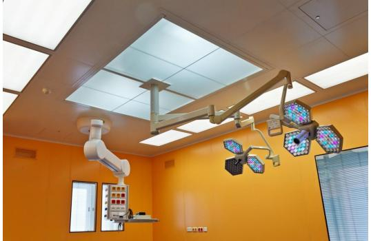
The laminar field is formed as a compact welded unit. Part of the laminar field are connection points for the ventilation ducts and a prepared installation chamber for the tube.
