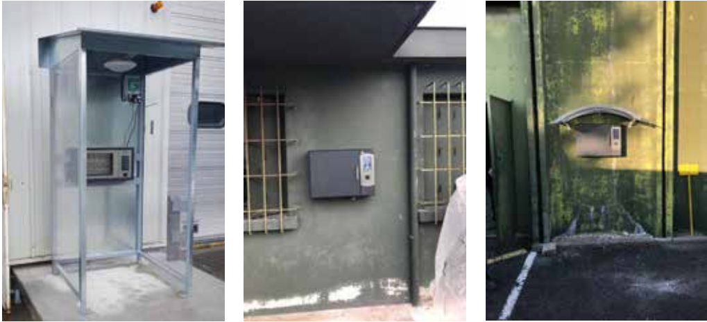
ecos key 20 and 40 in outdoor use at various military sites, each equipped with a cover to protect the user and system
