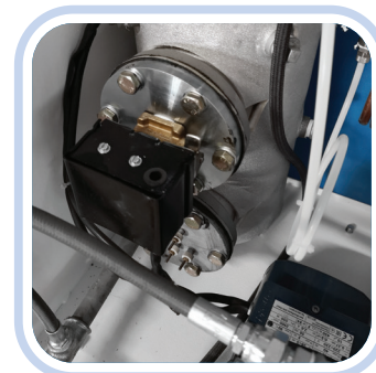
Controllo livello acqua in caldaia mediante galleggiante. Water level control in the boiler by means of a float.
