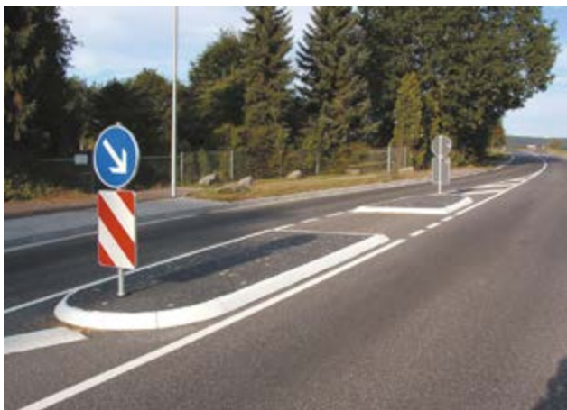
Angled kerbs adhered to asphalt with SILIKAL® R 17 mortar for a pedestrian crossing
