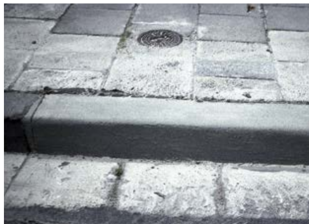
Renovation of kerbstones with SILIKAL® R 17 mortar
