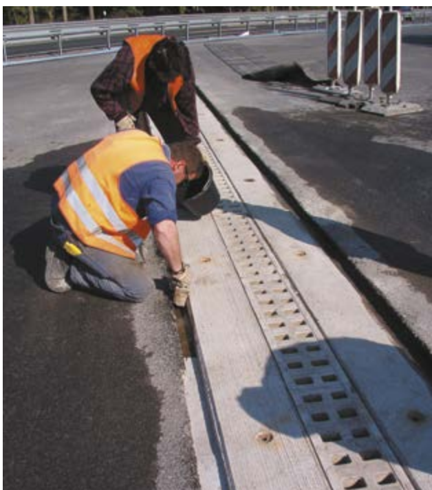
Installation of the lateral drainage channels in a motorway
