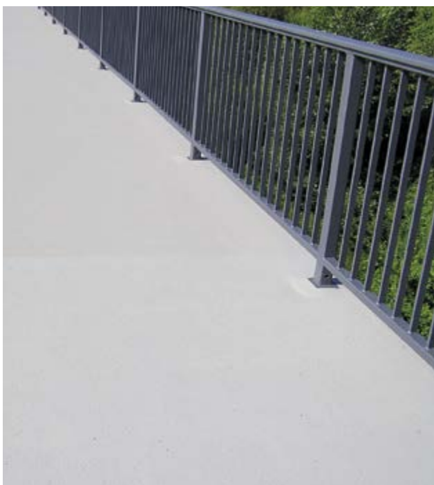
Bridge coating incl. handrail attachment
