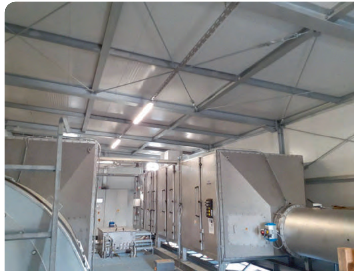
Two-filter systems for a total exhaust air volume of 60,000 m³ clean the odour-laden exhaust air and recover process waste heat. Photo: KMA Umwelttechnik
