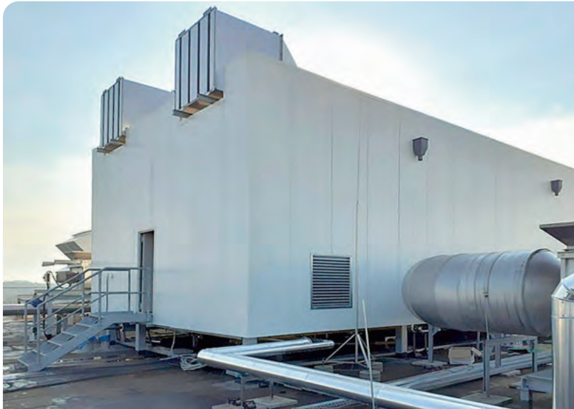
The central filter system is located in the weather protection housing on the roof. Photo: KMA Umwelttechnik
