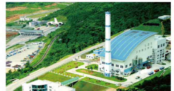
Shenzhen Nanshan Waste-to-Energy Plant
