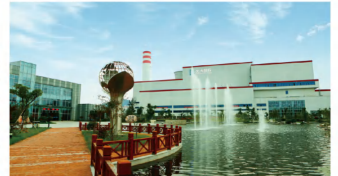
Everbright Environmental Protection Technology Co., Ltd. (Nanjing Waste-to-Energy Project)
