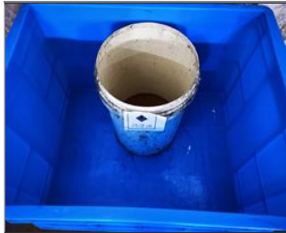
Photo of chemical storage room (if applicable) 3-1 Photo of secondary container for chemical.jpg
