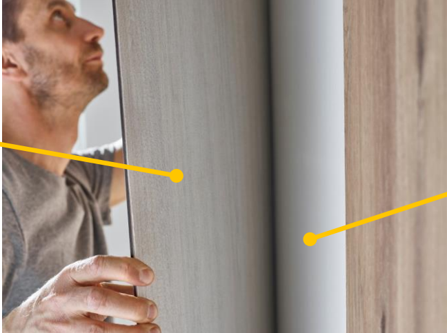
Gripping element with self-adhesive applied on the wall or on the floor
