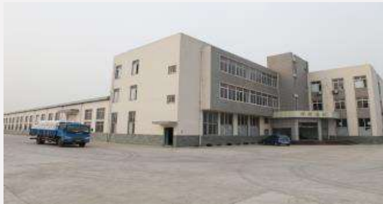
Filter media plant
