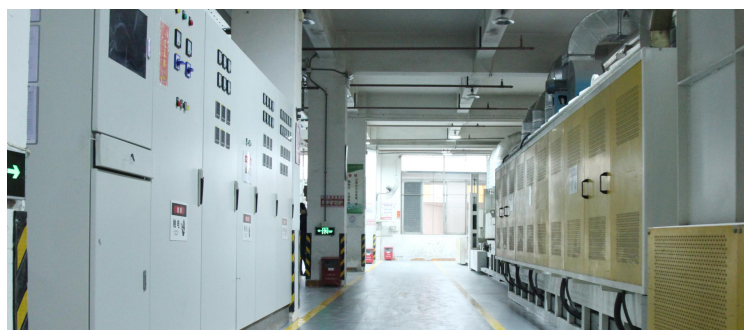
气氛保护铝连续钎焊炉 Atmosphere protected aluminum successive brazing furnace
