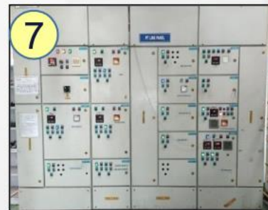
Auto-Control Panel <Conveyer Stop in Case Of Burnet trip & Temp out spec as required 148-150°C>
