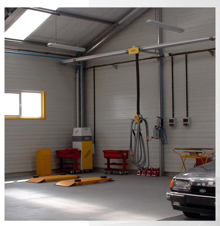
Extractors equipped with an high-performance sleeve-filtering system, an automatic or programmable cleaning-filter system. A control panel "touch screen" allows to monitor the functioning and regulate the cleaning ranges. High energy-saving guaranteed by a switching-on / off automatic system which starts the suction turbine when the first tool is switched on and turns off the turbine a few seconds after the switching-off of the last tool.
