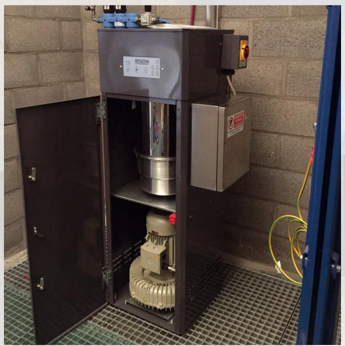
Stucchi 1950 ATEX extractors prevent the creation of static electricity, the motor overheating and other measures. All ATEX products of the Stucchi 1950 range respect and go beyond the security qualification imposed by the legislation, being always equipped with certified ATEX motors by the manufacturer.
