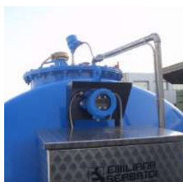
Electronic level gauge.
