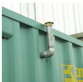
Tank's vent pipe
