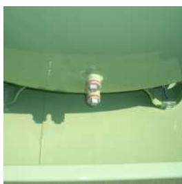
1" drainage point for routine maintenance and cleaning
