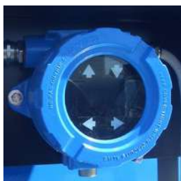
DIGIMAG level gauge (inox float).
