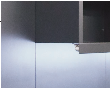
Extended front pelmet to allow fitting of lighting behind
