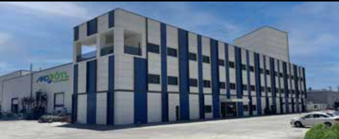
Ako Tyre Recycle Plant
