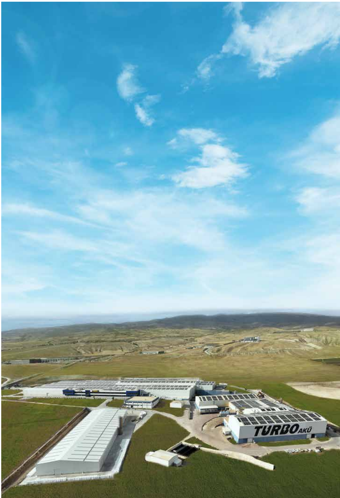
Ako Battery Factory
