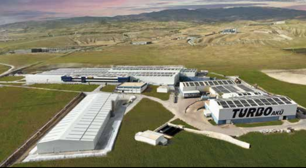
Ako Battery Factory
