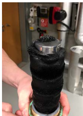
Inner view of a large version Ferro-Cleaner. Example of Ferro-Cleaner efficiency.
