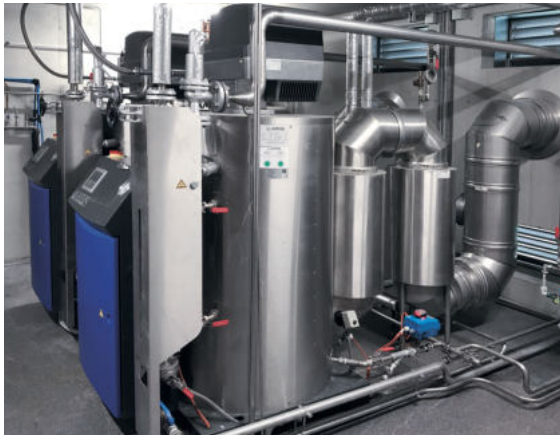
Fig.: Multiple unit steam system with second economiser on base frame
