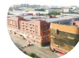
11 office and production buildings
