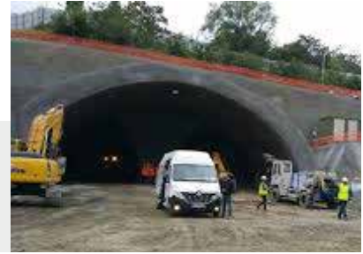
NORTH MARMARA TUNNELS
