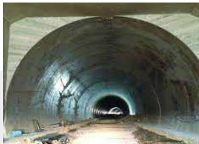
BOZTEPE & OCELI TUNNELS
