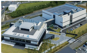
Takasago Thermal Engineering Innovation Center, Japan
