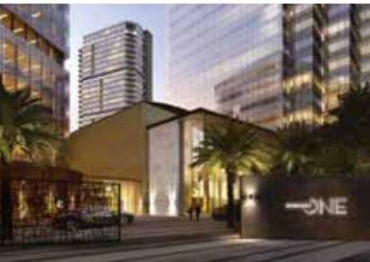
Four Seasons - Bangalore, India Turnkey Hot Water & Steam System
