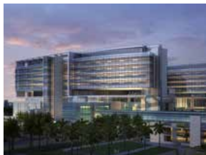
KSU - Riyadh, Saudi Arabia Turnkey Hot Water & Steam System
