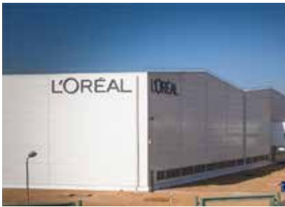
L'Oréal Cosmetics Plant - Cairo, Egypt Turnkey Hot Water & Steam System
