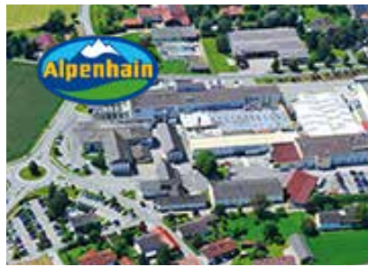
ALPENHAIN Camembert - Germany High Capacity Water Heaters
