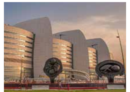
Sidra Med. & Research Center - Doha, Qatar Turnkey Hot Water & Steam System
