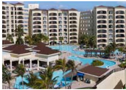
The Royal Caribbean - Cancun, Mexico Hot Water Boilers & Heat Exchangers
