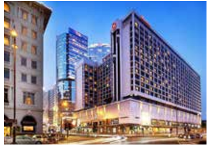
Sheraton Hotel & Towers - Hong Kong Turnkey Hot Water & Steam System
