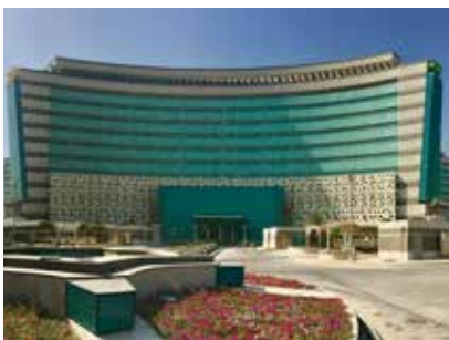
Sheikh Jaber Hospital - South Surra, Kuwait Turnkey Hot Water & Steam System
