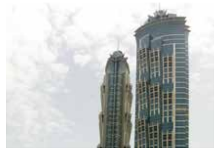
JW Marriott Marquis - Dubai, UAE Turnkey Hot Water System
