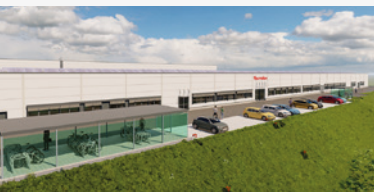
Production and Warehouse (11.000 m 2 ) in Bischoffen
