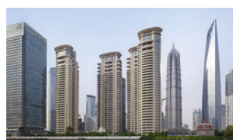
Tomson Riviera Apartment Towers Shanghai, China
