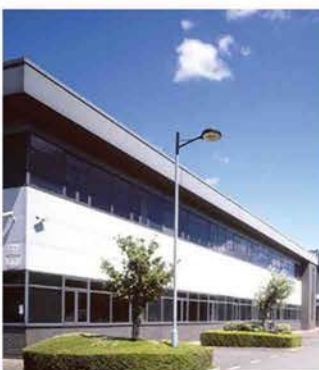
Redhill Data Centre. Redhill. Great Britain.
