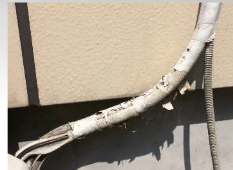
Insulation without UV protection damaged by solar UV exposure
