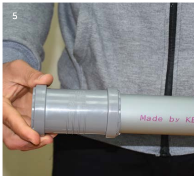
Jointing (push the spigot end into the socket until it's fully in place)
