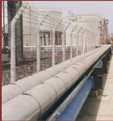
12 Kms of Thermotrace Self Regulating Tracer installed at Indian Oil Corporation Ltd. Panipat (operational since 2006)
