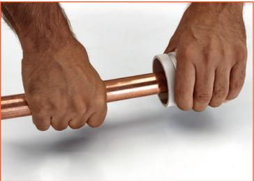
2) **Carefully deburr the pipe**, both internally and externally, as a possible residual burr could damage the O-rings and compromise the tightness of the connection.
