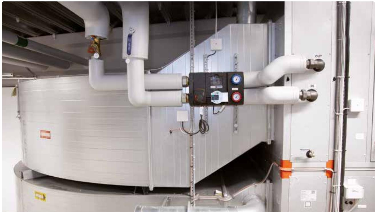
A circulation unit with a 3-point actuator which, in combination with the special valve regulation, provides unique stability, high controllability and precision when regulating.
