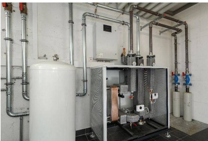
Figure 2 (PR_ISH_MegapressS_EN_202503): For the secondary connection of compact heating systems, Viega offers the "Megapress S" press connector system, which can withstand high thermal loads and can also be pressed with the steel pipes typically used in district heating networks. (Photo: Viega)
