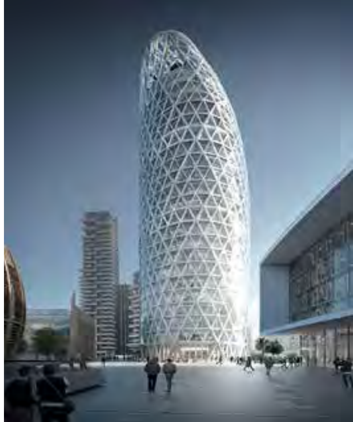
TORRE UNIPOLSAI - MILANO ITALY - 2023 - Central heating/cooling
