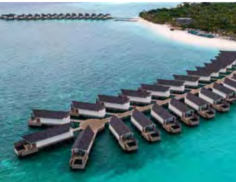
OZO RESORT - KUDAKURUTHU MALDIVES - 2021 - Water supply system
