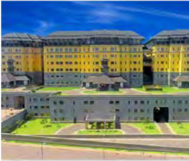
DIFENCE HEADQUARTERS – AKUREGODA COLOMBO – 2021 Heating/cooling system
